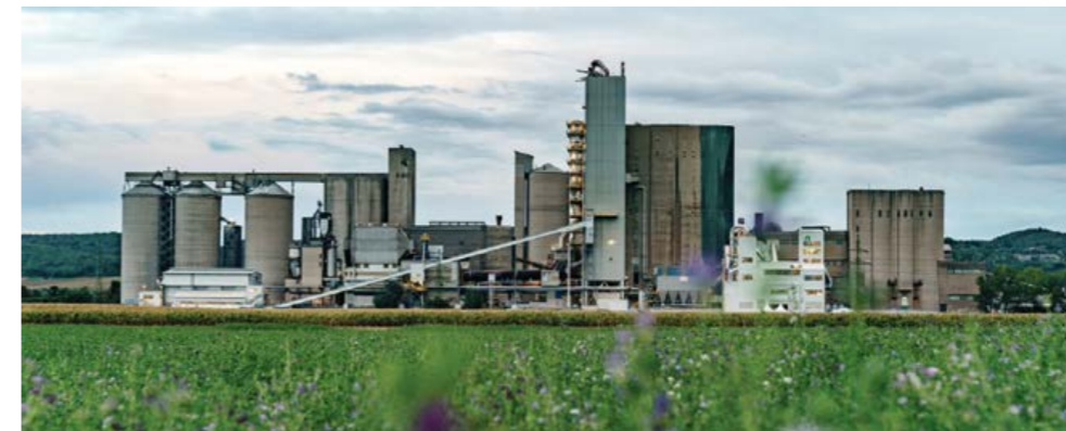
Holcim Werk in Mannersdorf
