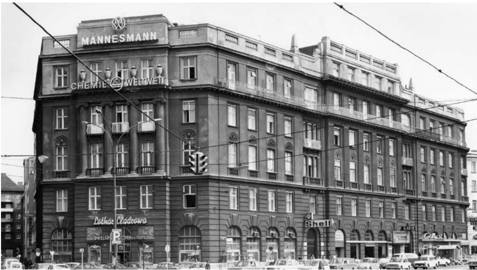
Schwarzenbergplatz 8 in the 3 rd District in Vienna (©Photo archive - Federal Monuments Office)
