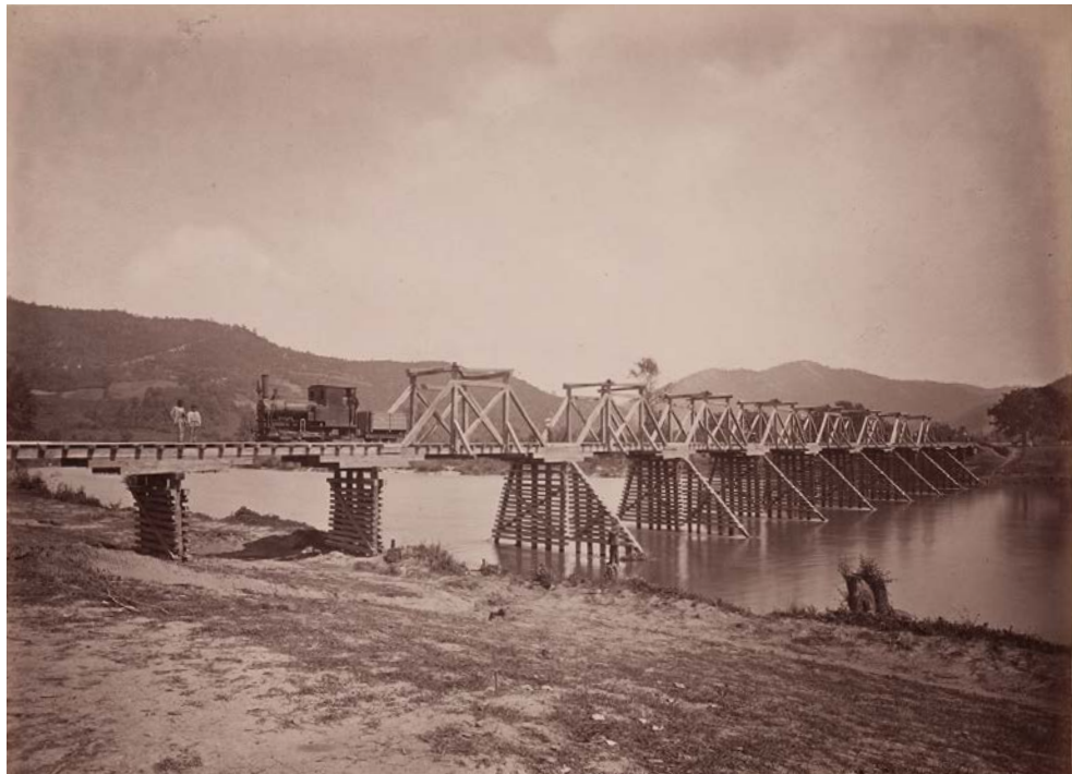
Jelacic Bridge near Maglaj, Bosnia-Herzegovina, 1880 (©Austrian National Library)
